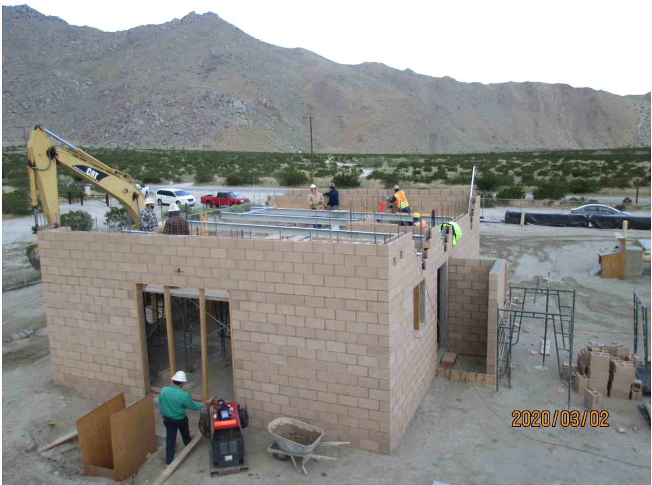
Photo 1: The contractor setting the I-beams in the building.
