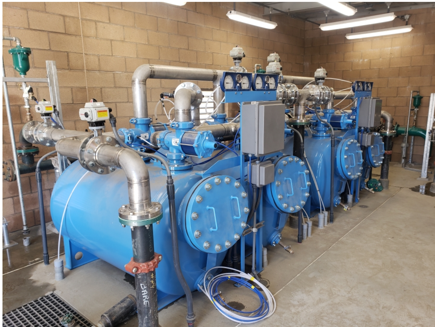
Photo 6: The filters installed in the filtration plant.
