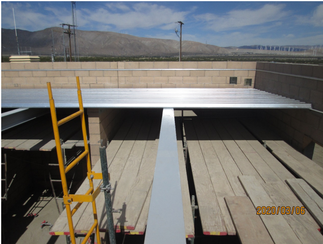
Photo 3: The I-beams and a section of the metal roofing.
