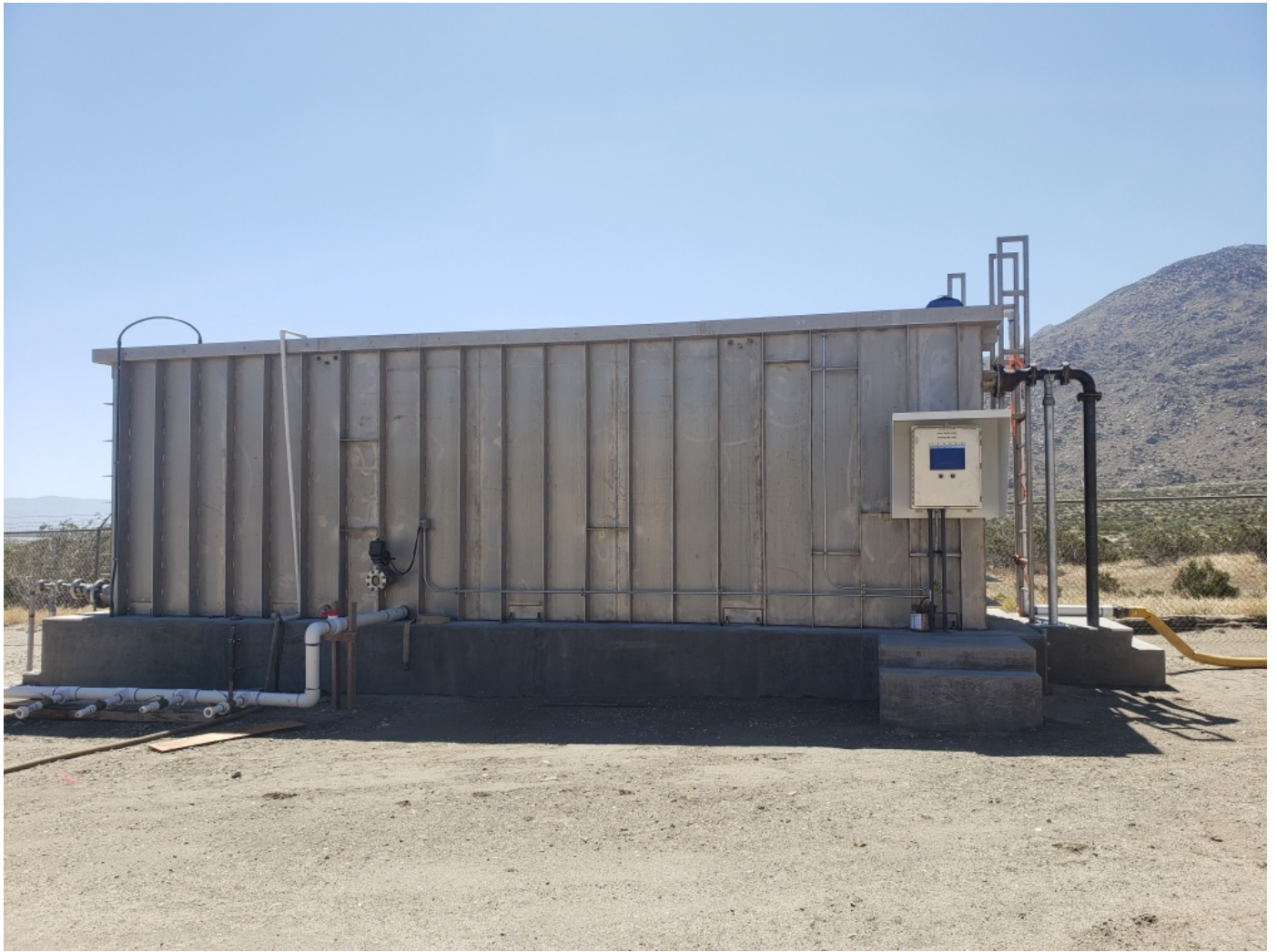
Photo 8: The backwash and rinse water clarifier. Note: Per the plans, the final grade will be raised.
