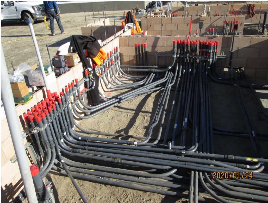
Photo 5: The sub-grade beneath the control room. An array of conduit are installed to connect the various components together to operate the plant and filters.
