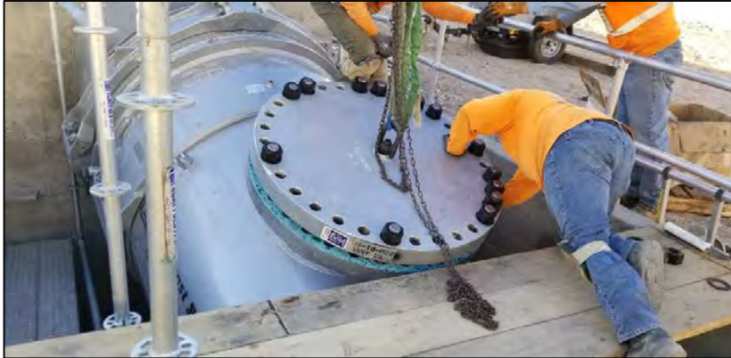
Blind flange installation at Iron
