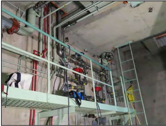
Completed C/W piping at Hinds
