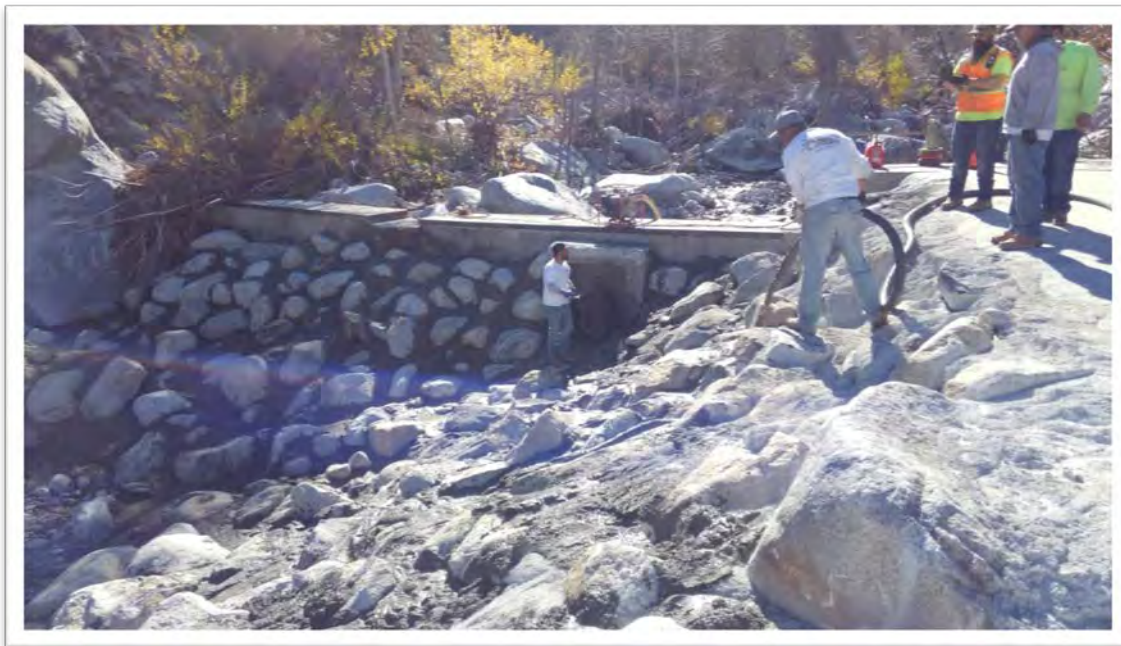
Photo 3: Below the Snow Creek Diversion after the repair work. Contractor is pouring slurry to lock the rocks in place.
