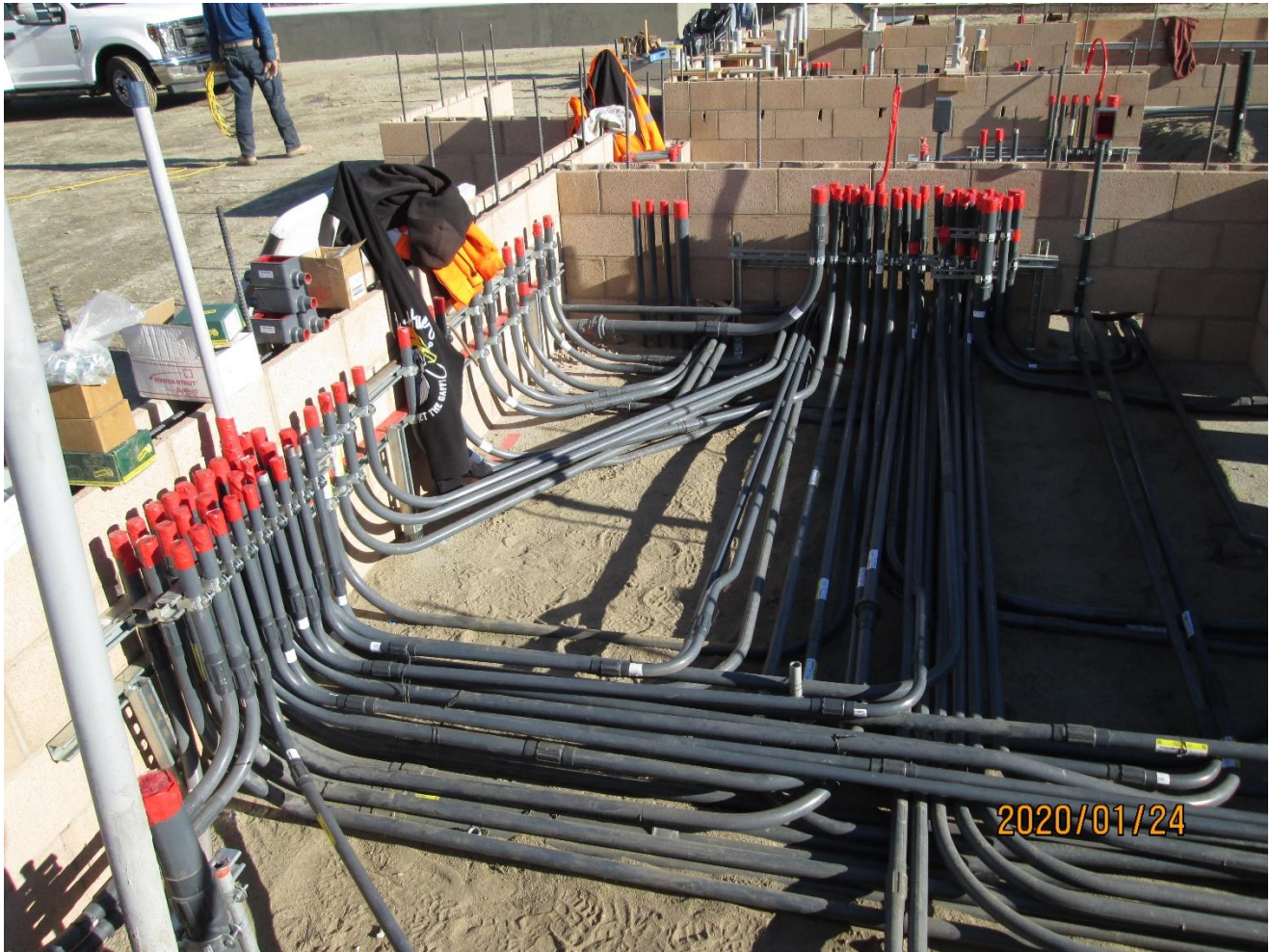
Photo 4: The sub-grade beneath the control room. An array of conduit are installed to connect the various components together to operate the plant and filters.
