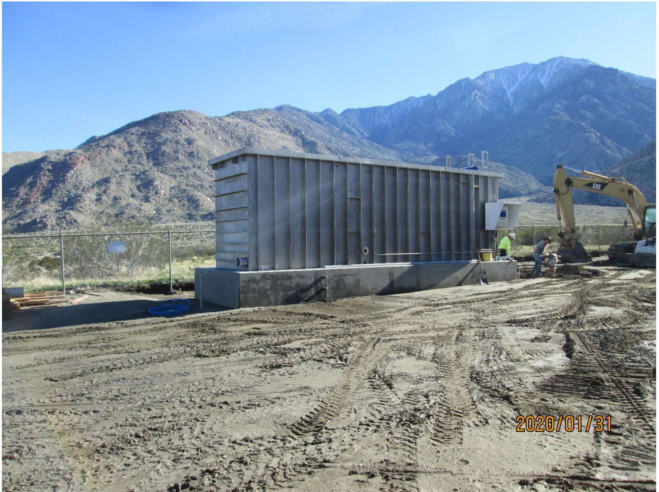
Photo 5: The backwash and rinse water clarifier. Backwash and rinse water will be diverted to this unit where any fine sediment will be removed. The clarified water will be returned to the filters. Without the clarifier, the backwash and rinse water would need to be handled onsite or hauled/piped offsite.
