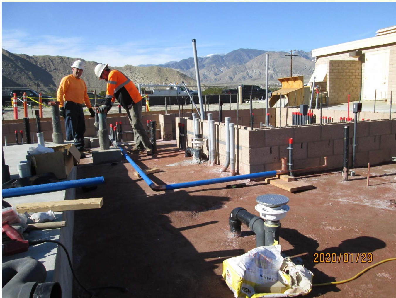
Photo 3: The sub-grade of the filter room. The extensive array of piping and conduit required multiple layers to complete the installation. The lower level of conduit and pipe was backfilled with concrete slurry to ensure proper compaction around the lower pipes and conduits. This level will be backfilled with slurry prior to the final reinforced concrete floor being placed.
