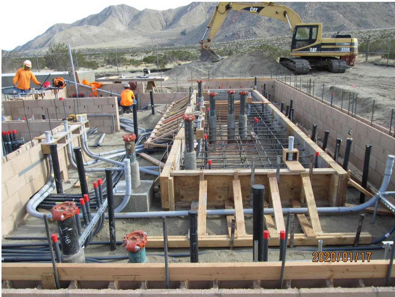
Photo 2: The sub-grade of the filter room. The proposed filters will sit on a reinforced foundation. The filters are connected by an array of electrical conduit, potable water pipes, raw water pipes, and drain lines.
