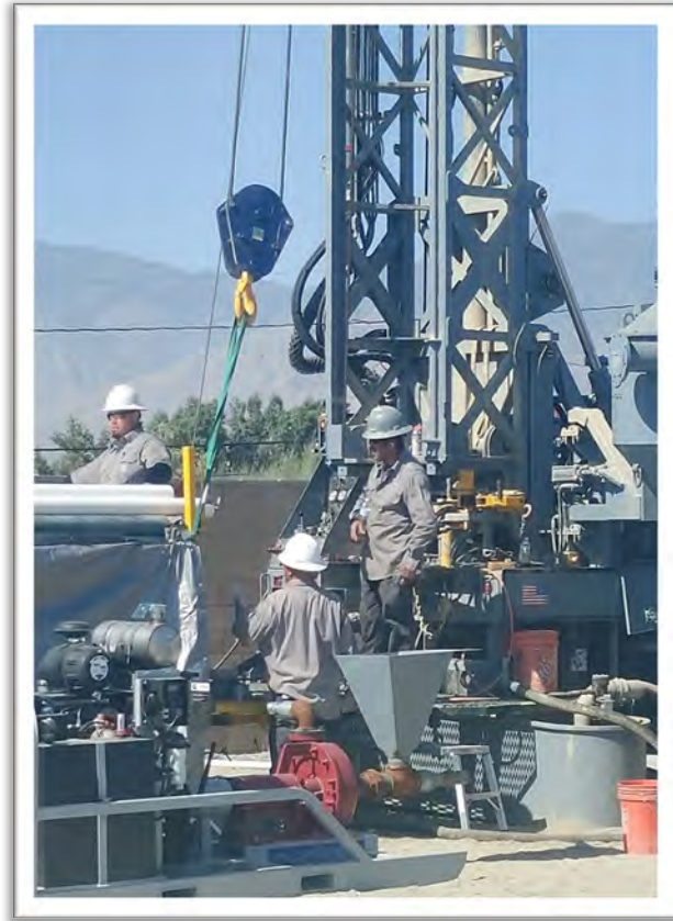
Installation of tremie pipe and well casing
