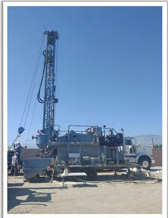
Installation of tremie pipe and well casing
