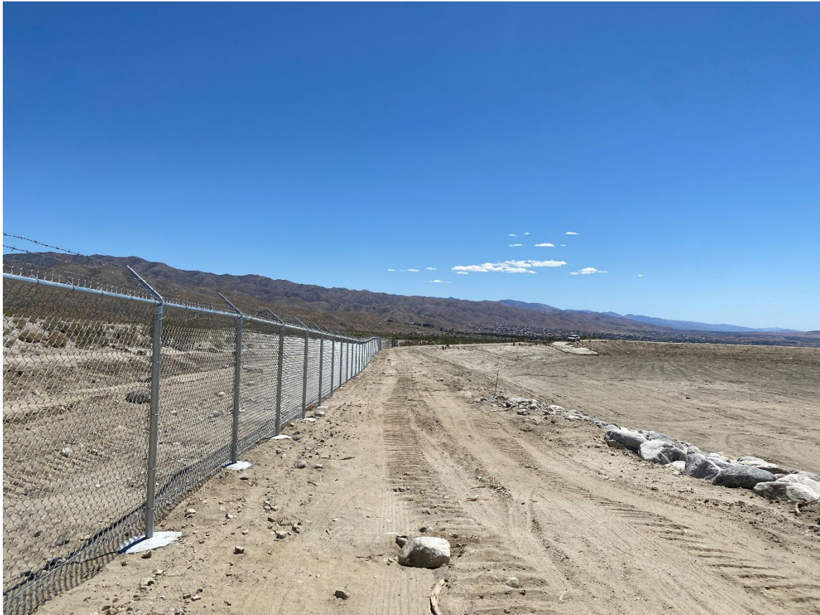
Photo 6: Fence on North Side of Debris Basin Looking East.
