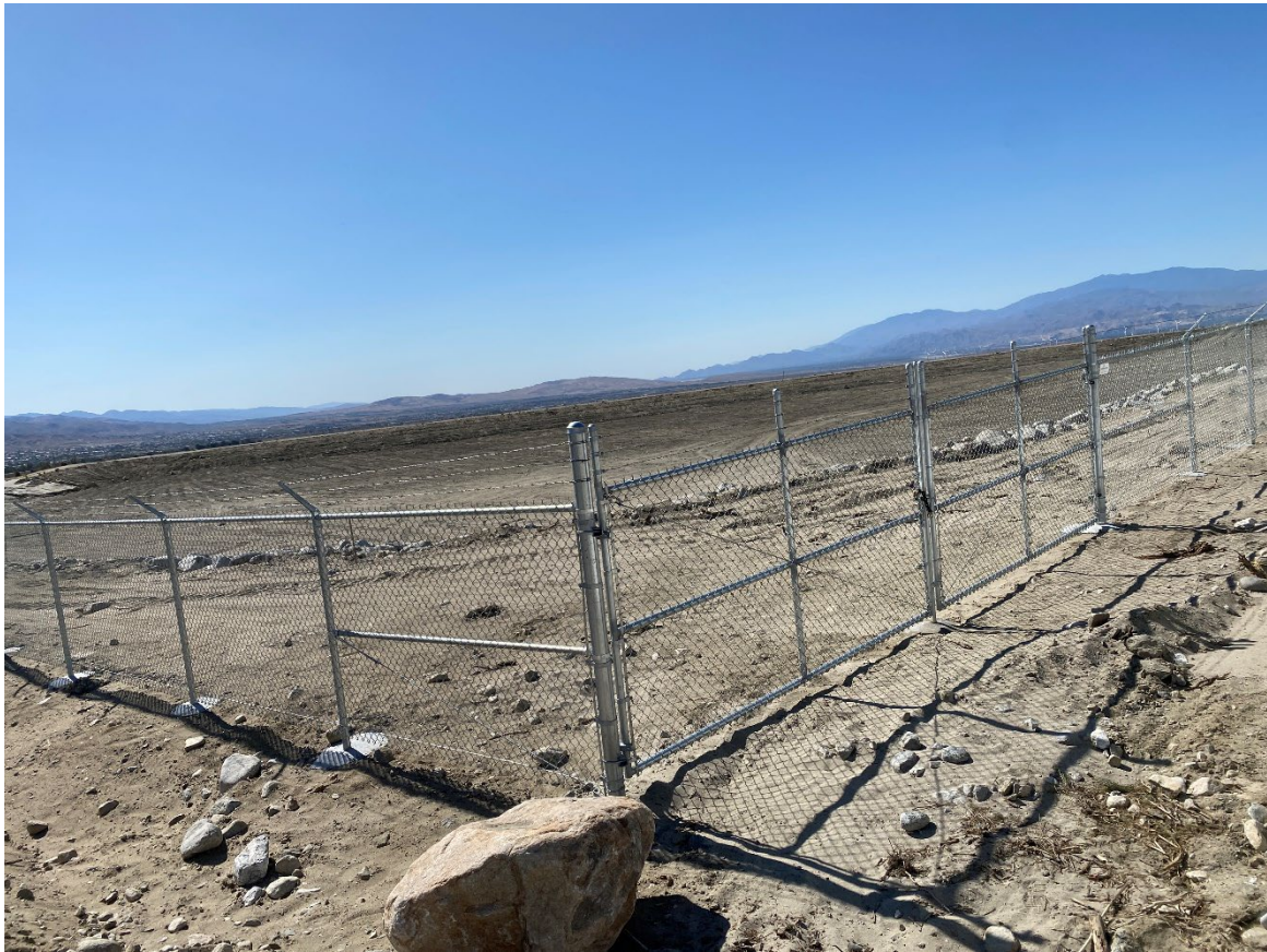
Photo 5: Fence at Northwest Corner of Debris Basin Looking Southeast.
