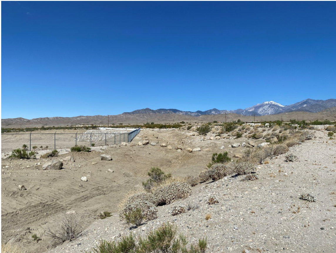
Photo 3: Mission Creek Overflow Channel Looking West.
