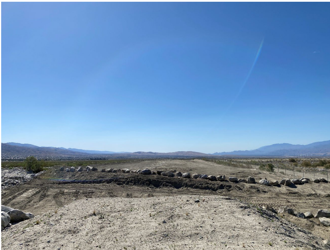
Photo 4: North Levee Looking Southeast.
