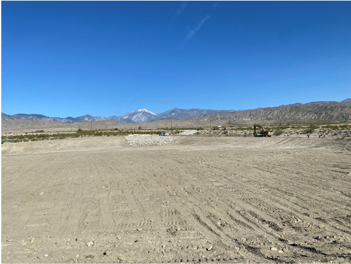
Photo 1: Cleared Debris Basin Looking West.
