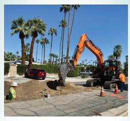
Desert Water Agency is replacing several aging water pipelines throughout our system to help improve water reliability, lower repair costs and reduce water loss.
