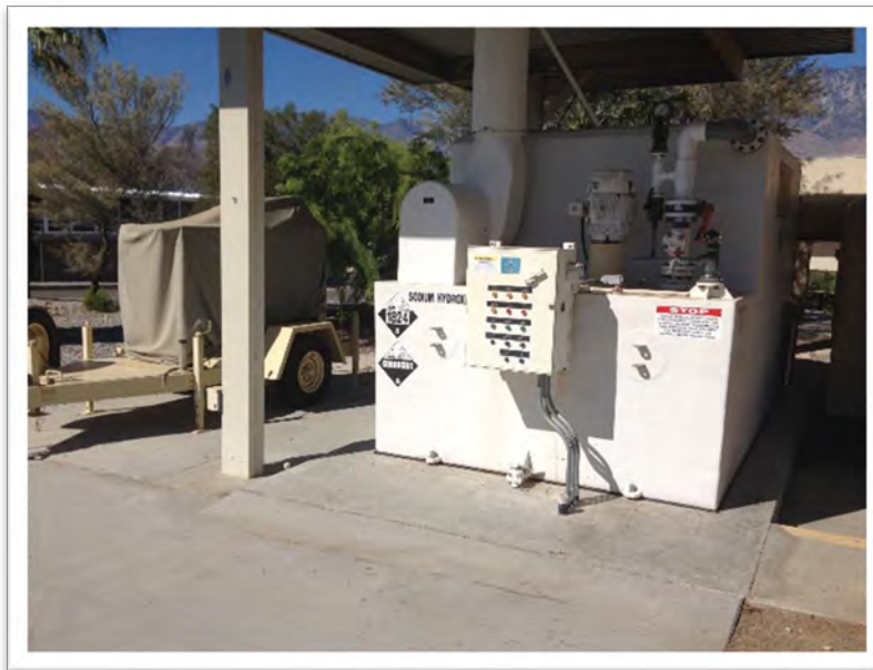
Photo 1: The original Caustic Soda Liquid Scrubber.
