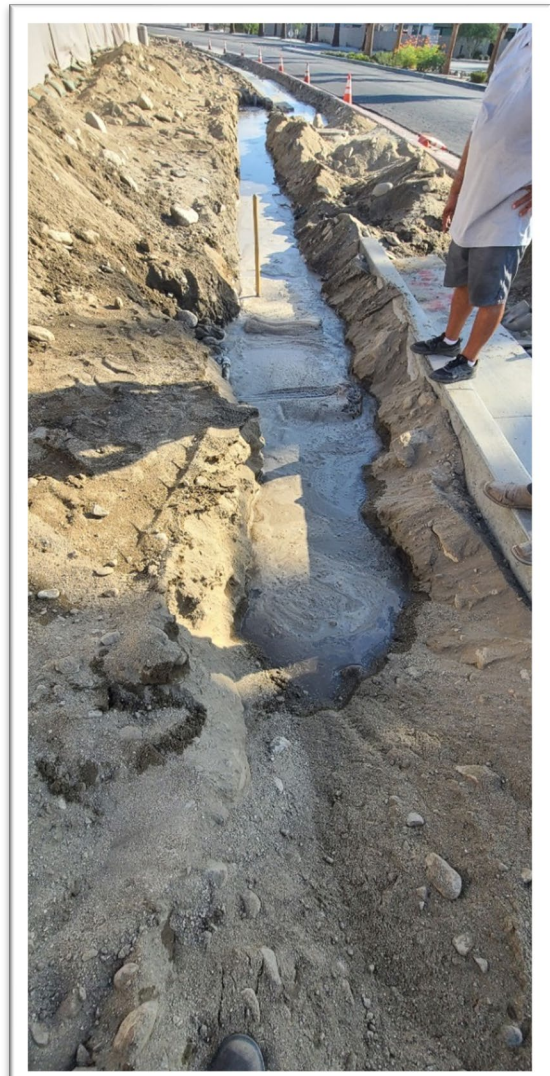
Trench that they were installing conduit and hit our service.
