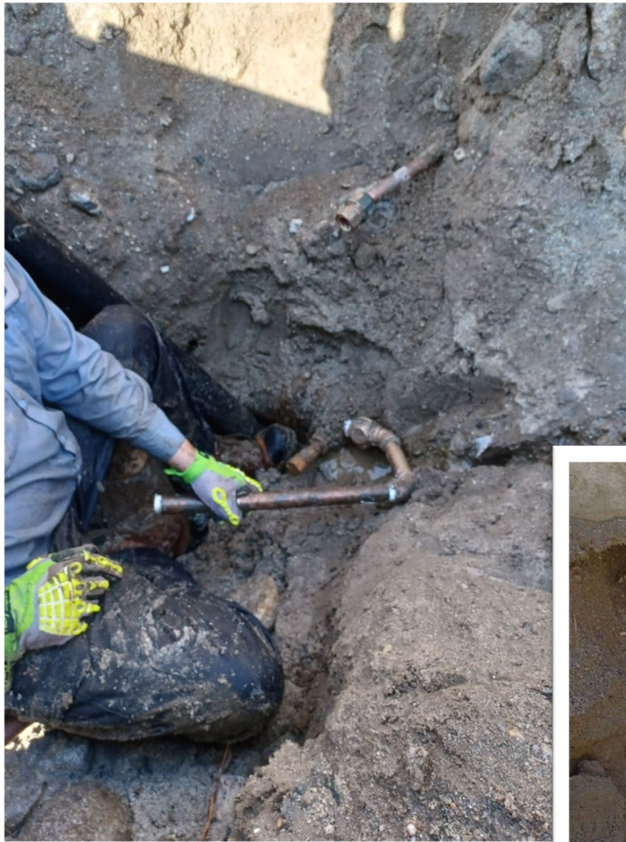
Picture of the corp stop that broke at the threads going into the saddle.
