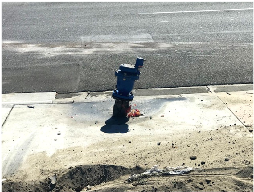
Damaged air-vac.
