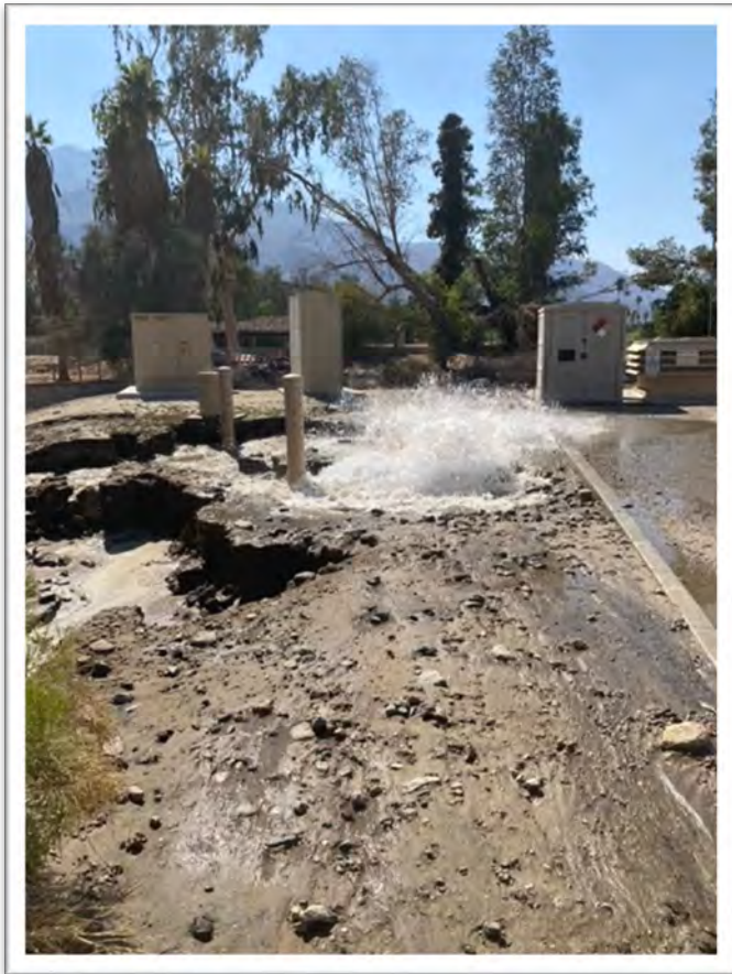
Figure 1: Water discharging from the Flow Meter Vault. Significant erosion occurred as a result of the discharge.
