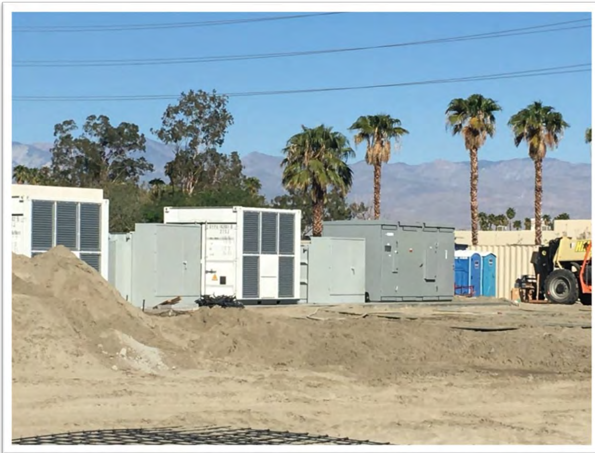
Photo of inverters (white), transformers (light gray), and switchgear (darker gray)
