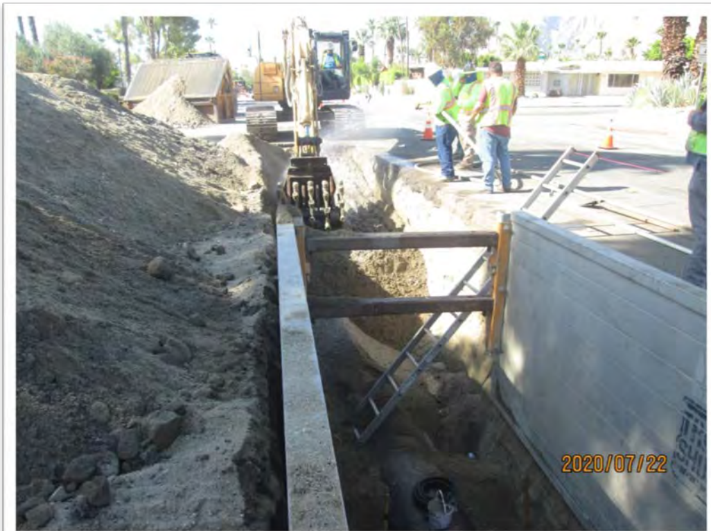
Photo 3: Jones Brothers Construction backfilling the 30" Ductile Iron Pipe on Avenida Caballeros.
