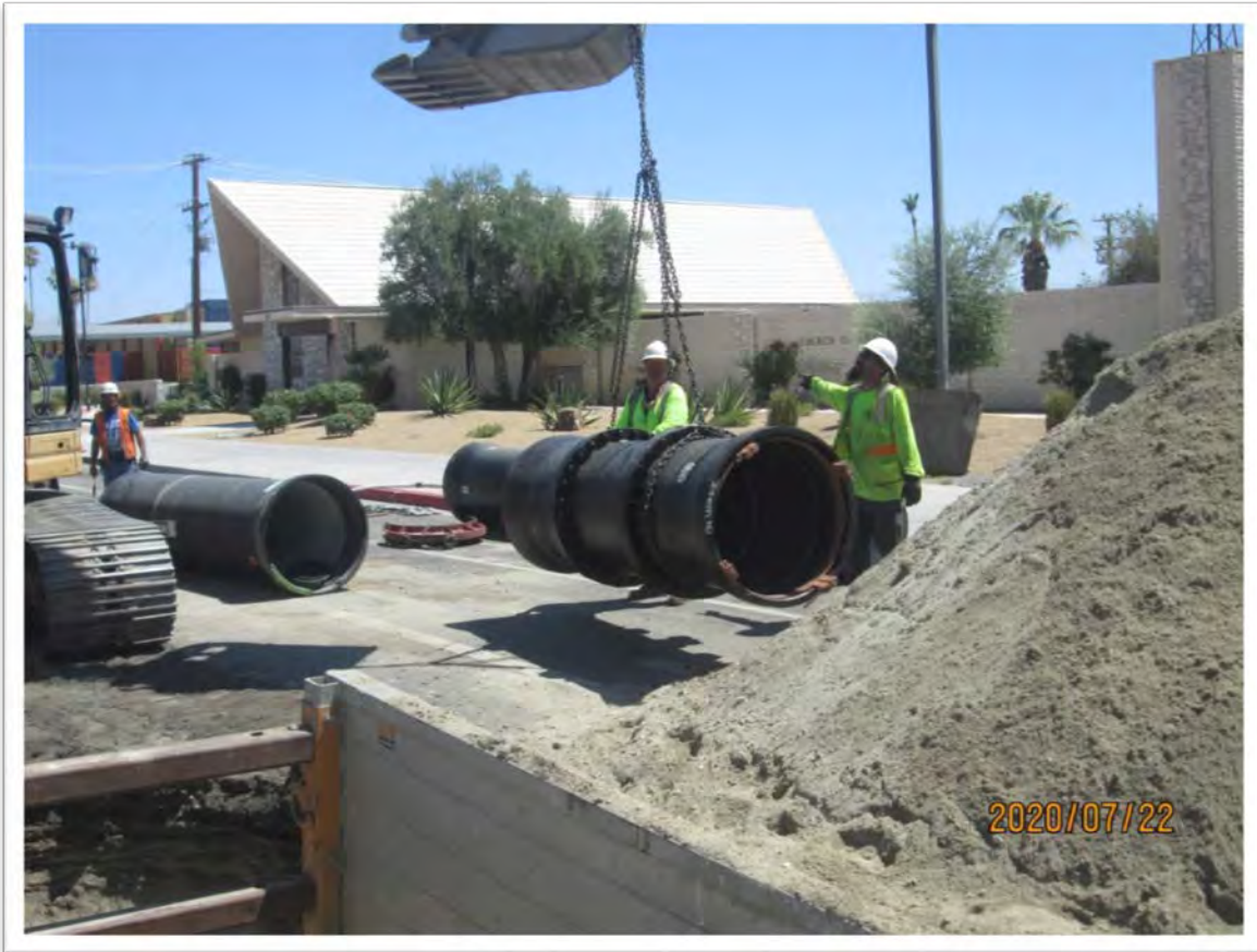
Photo 1: Jones Brothers Construction preparing to install 30" Ductile Iron Pipe on Avenida Caballeros.
