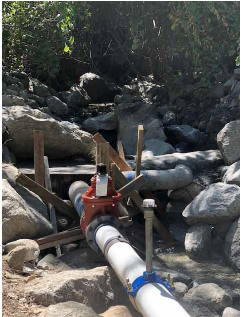
Photo 5: Intake pipe repair
