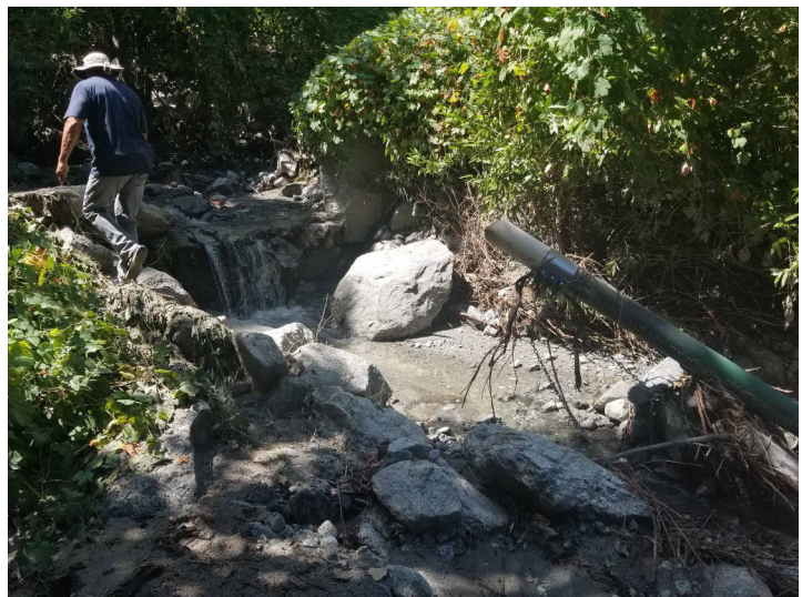
Photo 2: Intake piping damage after storm
