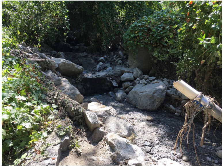
Photo 4: Cleaned intake with damaged pipeline
