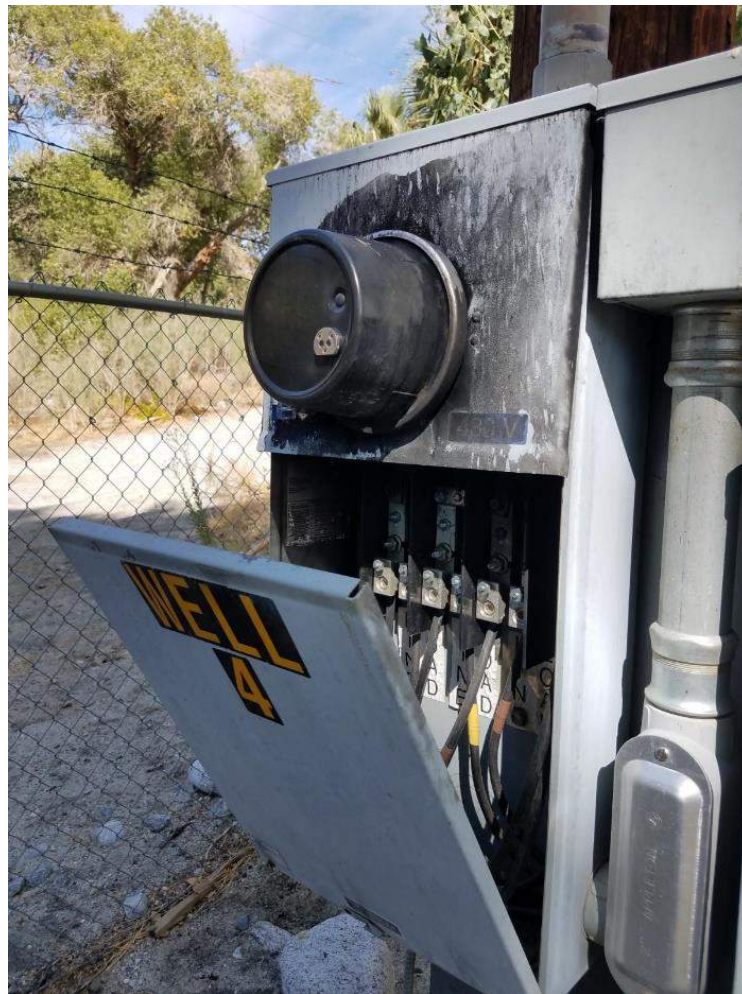
Photo 2: The Edison Meter for the 4" Pump.
