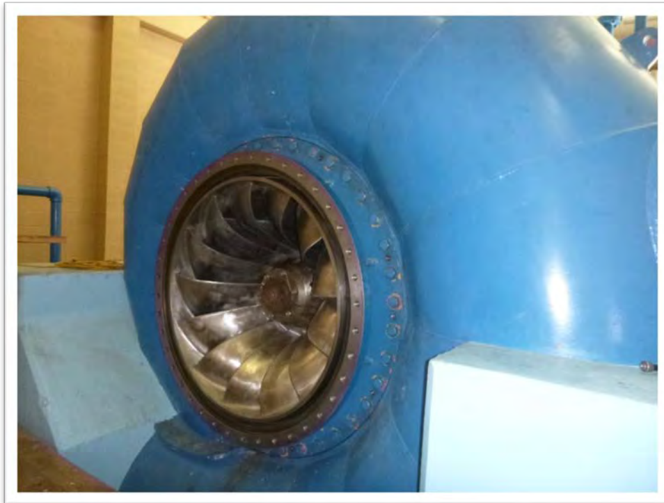
Photo 2: The runner was re-welded to original factory specifications.
