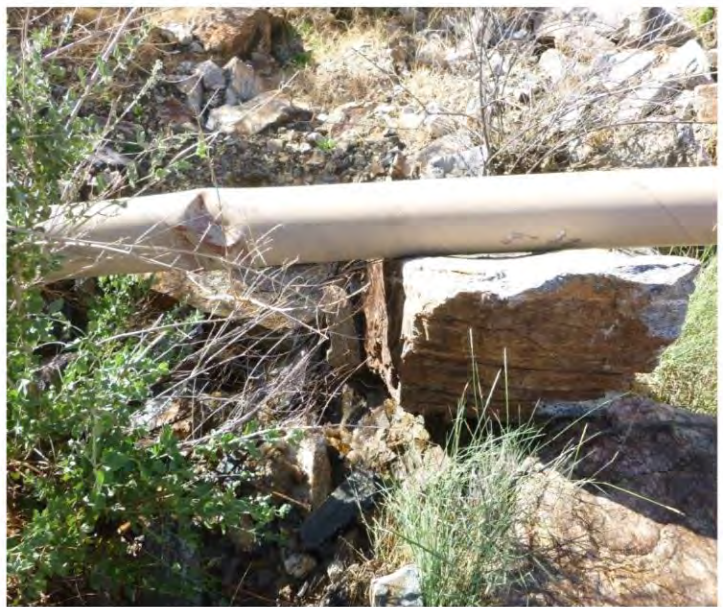
Photo 2: The boulder that damaged the pipe.
