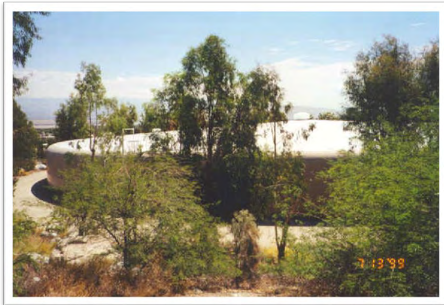
Palm Springs Reservoir No. 2. Reservoir is 232 feet in diameter and 40 feet tall (approximately ½ is buried belowground). When full, the reservoir holds 12 million gallons of water.
