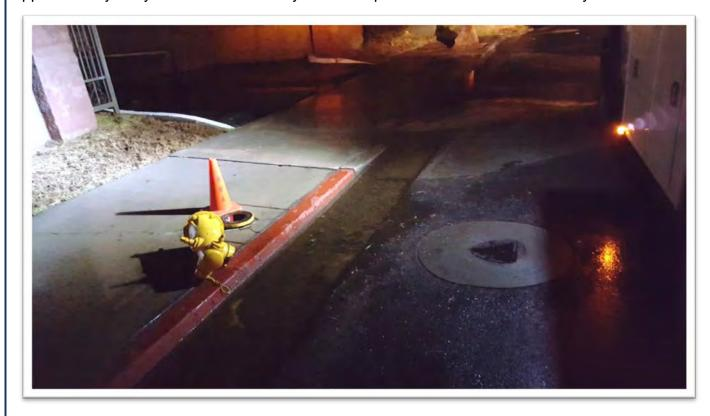
On January 12 at approximately 6:00 p.m. stand-by responded to hit fire hydrant on Arenas Dr. and Saturmino Dr. This was a hit and run. Staff was unable to access the fire hydrant valve and had to shut down the main line. They were able to reinstall the fire hydrant and put it back in service. A police report was made. The water loss was for approximately one hour through a fully open 6 inch fire hydrant bury.
