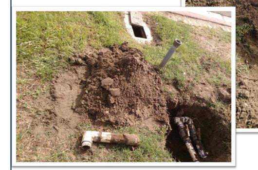
On August 12 at approximately 8:00 a.m., staff responded to a hit angle stop by a bobcat tractor at 3099 Linea Terrace. Staff replaced the angle stop and the meter register. A damage report was filled out and the developer Alta Verde Group will be charged. The water loss was from a broken meter coupling on the angle stop which ran for approximately 5 minutes.
