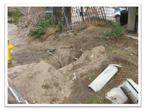
On April 10 at approximately 10:00 p.m., stand-by responded to a hit four inch air-vac on Hwy. 111 on the Snow Creek line. Staff shut the air-vac valve off. There was no water loss. A police report was made. Repairs were made and the air-vac is back in service.
