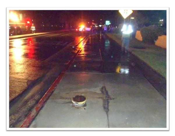
On March 18 at approximately 1:50 p.m. construction responded to a hit fire hydrant on the North West corner of Camino Centro and Vereda Del Sur. This was a hit and run. Staff was able to replace the bolts and gasket and put the fire hydrant back into service. The water loss was through a six inch opening for approximately 20 minutes. A police report was filed.
