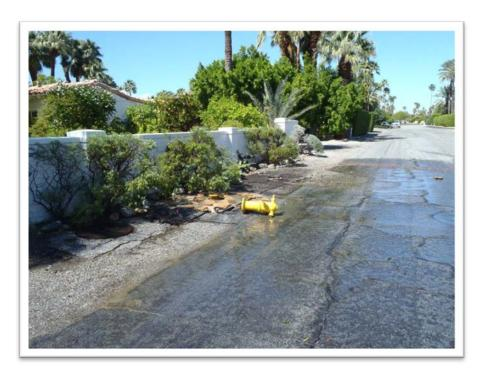
On March 30 at approximately 1:40 p.m. staff responded to a hit fire hydrant at 67555 East Palm Canyon Drive (this was a hit and run). The fire hydrant had to be replaced and is back in service. A police report was made. The water loss was through a fully open 6 inch opening which ran for approximately 20 minutes.
