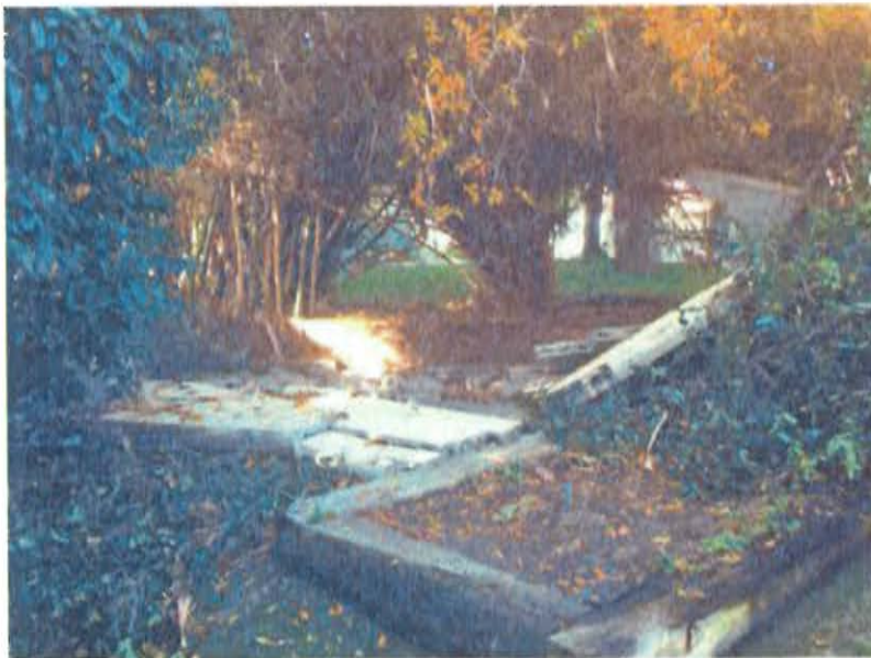
Left: Water ran thru front yard of 447 heading east to property line block wall. It then ran south along the wall until the force broke thru the wall and the water flooded into the Breimer property at 423. The property line block wall is lined on the Breimer side with a Carolina Cherry hedge which is approximately 20+ feet high. Broken portions of the block wall currently lay across approximately 10-15 Carolina Cherry trees which will need to be replaced as well as on top of the Breimer herb garden.
