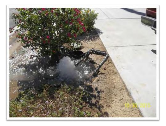
On November 2 at 9:00 a.m., staff responded to a two-inch service that was hit by contractors working for Alta Verde builders on Bogert Trail at the Linea tract. Staff made the repairs and put the service back in. The water loss was from a two-inch fully open for approximately thirty minutes. A damage report was filled out.
