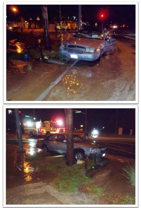
On October 7 at approximately 11:30 a.m., construction responded to a hit air vac by a contractor working at the Fashion Plaza (Palm Canyon Drive, South of Andreas Rd.). Staff made the necessary repairs, put the air vac back in service and filled out a damage report. The water ran from a fully open 2-inch riser for about 20 minutes.
