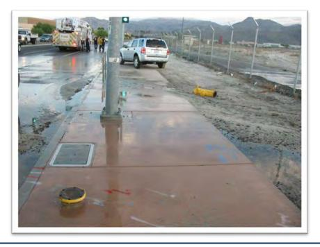
The Snow Creek Village alternate water supply is now in place. Construction, Engineering and Operations teamed up to make this supply viable. Staff used existing facilities with modifications to reverse normal flow conditions in order to make groundwater from the Palm Oasis area deliverable to the Village. Total capital cost was about \$55,000. In future fiscal years, improvements can be made to make alternative supply facilities permanent.
