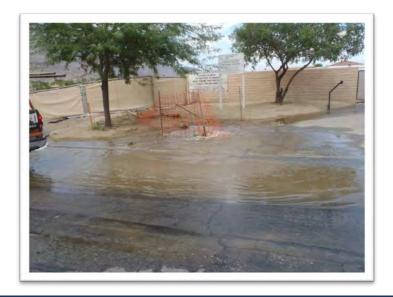
On September 10 at approximately 6:25 p.m. Stand-by responded to a hit fire hydrant on the west side of the intersection of Gene Autry Trail and Mission Road. A police report was made. The water loss was a fully open six inch riser that ran for approximately thirty minutes. The bolts and gaskets were replaced and the fire hydrant was put back in service.
